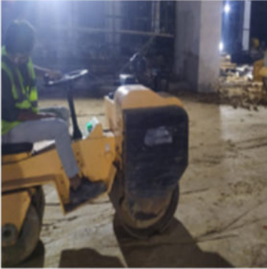
Fig. 1. Mini vibratory roller for compacting soft compressible strata.
