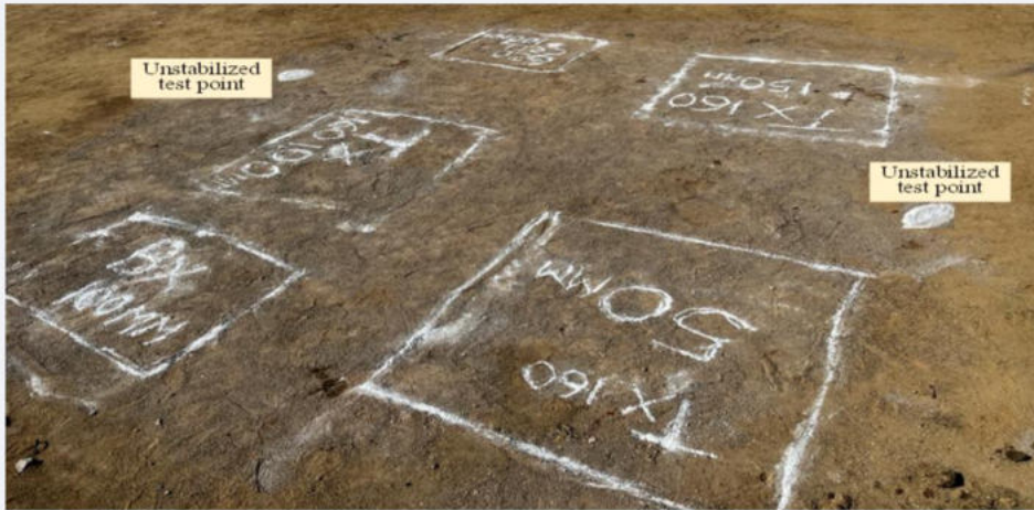
Fig. 6. Unstabilized and geosynthetic stabilized sections
